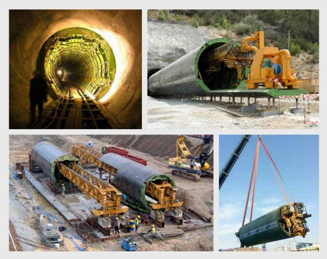
Telescopic and multi-section formwork for continuous "slipforming" or step by step concreting pours. Self-launching forms to operate in all slopes conditions. Fully mechanized movements integrated with automatic concreting system.
