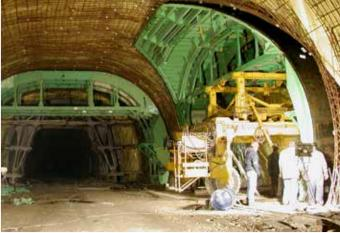
LAY-BAY TUNNEL AND CAVERNS Steel forms for widening and large-size caverns to be moved by special advanced traveller on rails or tyred traveller.
